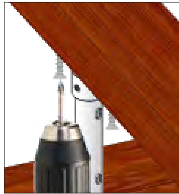
Figure BC. (LEFT) Attach the top of the stair stabilizer to the underside of the top rail with (2) two 1/4 x 2" flat head wood screws.
