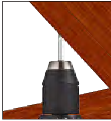
Figure BA. (LEFT) Drill pilot holes at the pencil marks in the bottom side of the handrail.
