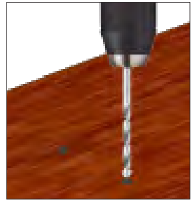
Figure BA. (LEFT) Drill pilot holes at the pencil marks in the bottom side of the handrail.
