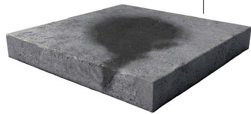
Untreated Concrete, Showing Water Intrusion
